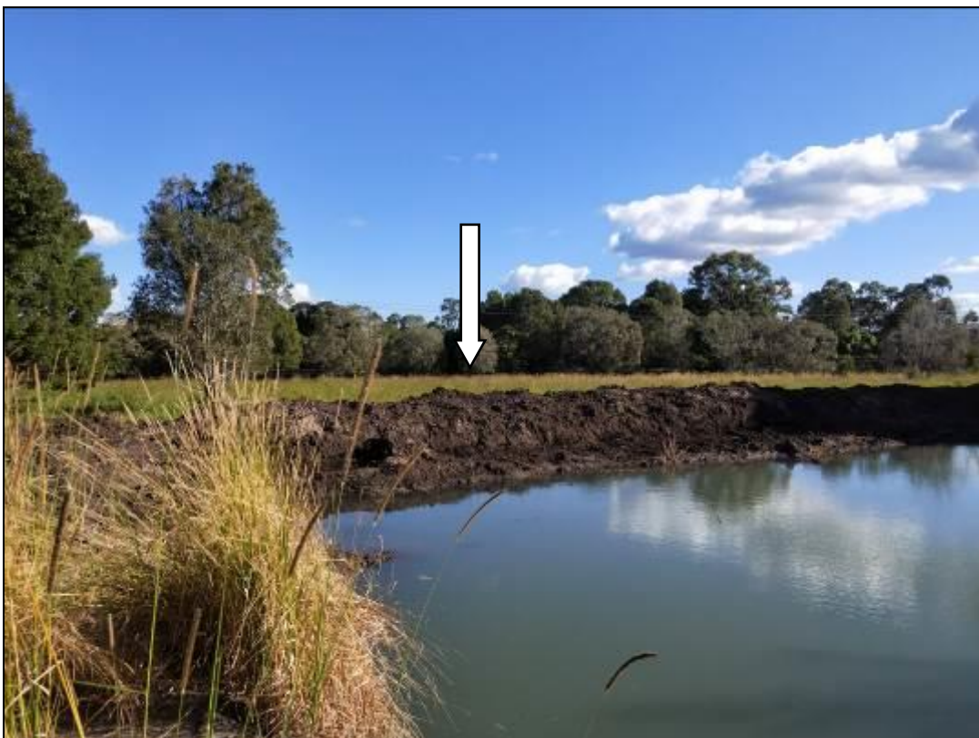
Photo 4 View S showing bunded watercourse (dam), proposed LAA downslope marked by arrow.
